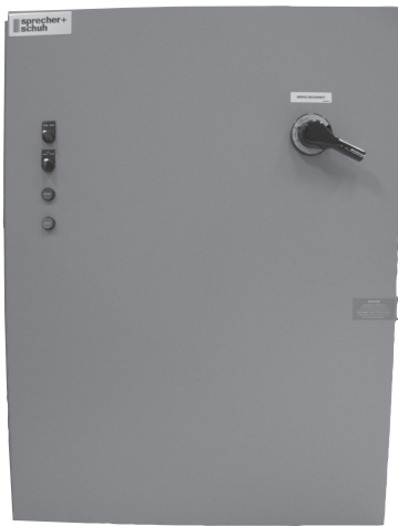
PFS Softstarter UL508A Service Entrance Custom Panel 150HP@480V AC
